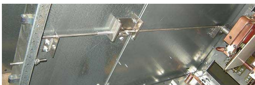
Figure 28 Interlocking device: Earthing switch and cable compartment door
