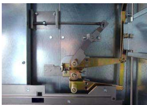
Figure 29 Interlocking device: Cable compartment door open preventing the DOU to be racked in
