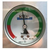
Figure 15: Gas pressure monitor
