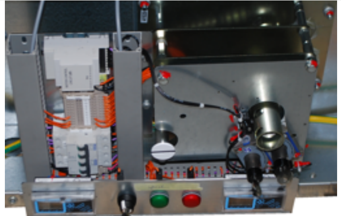
Motor driver integrated in motorized LBS drive for DF-2 cubicles.
