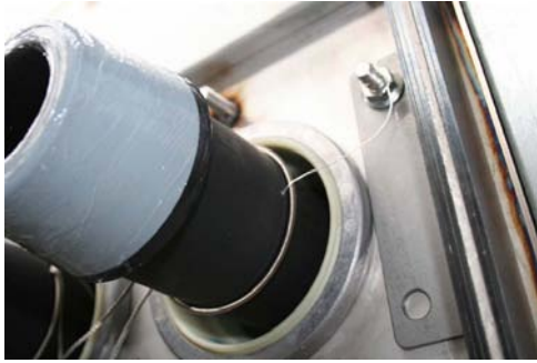
Figure 13: Ground connection
