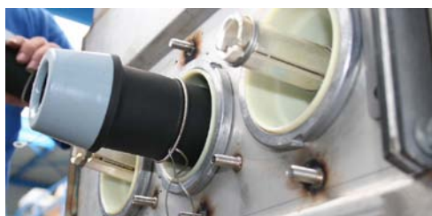
Figure 12: Busbar insulation mounted
